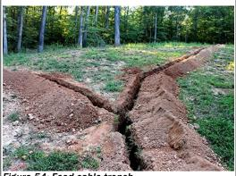
Figure 54: Feed cable trench
