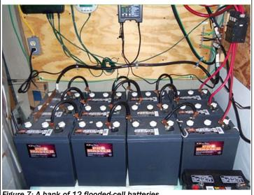
Figure 7: A bank of 12 flooded-cell batteries
