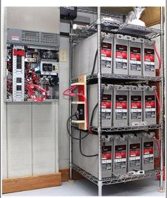
Figure 63: Battery rack
