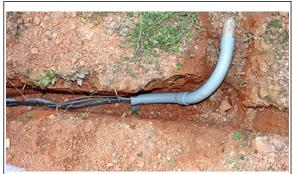
Figure 42: Feed cable conduit into house
