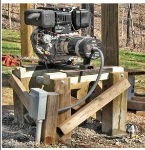
Figure 60: 6.5 KW diesel generator
