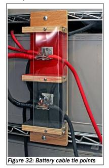
negative (black cable) tie bar is barely visible in the upper-right corner of Figure 7. This one is fabricated from heavy copper bar with holes for large bolts to hold the terminal lugs.
