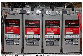
Figure 6: String of four AGM batteries
